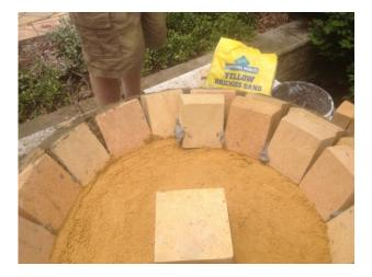
Using the airset mortar keep doing your 4-5mm internal mortar joints and fondu in between to lock the rear in and strengthen it.
