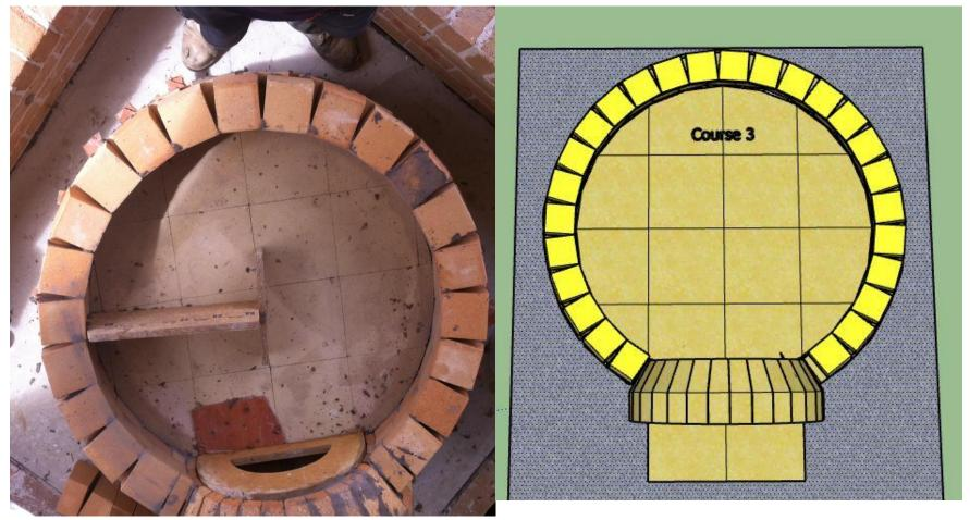
Using the chamber template as a guide from the centre of the oven rotate it around and lay your bricks in the pattern for the second layer Make sure you lean the bricks against the template guide to correctly set the angle
