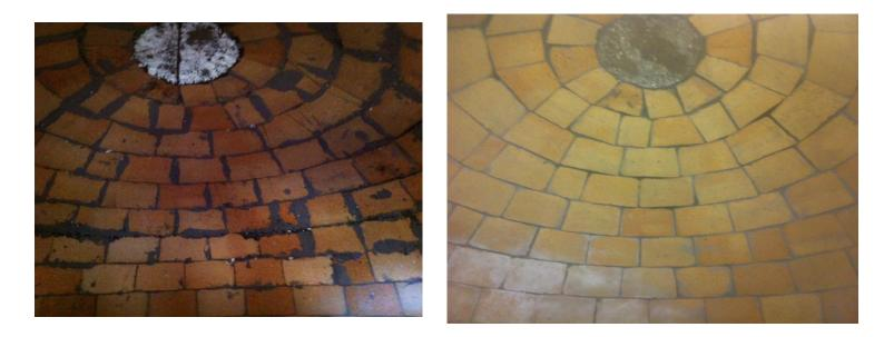
After leaving the sand plug in overnight (even longer for colder conditions) moisture free, Gently knock the bricks out holding the timber template in place. Start with the 2 front and then do the rear. Clean the sand out and any debris and you should be left with the top left picture. You will have to venture inside the oven to clean the internal jonts using a DAMP But not wet sponge. Too much water can cause weakeness in the mortar.
