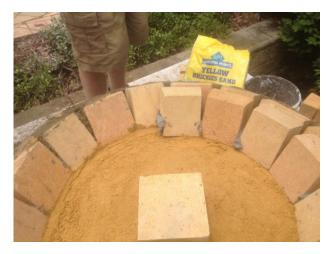
Using the airset mortar keep doing your 4-5mm internal mortar joints and fondu in between to lock the rear in and strengthen it. Follow the notches on the template for each row
