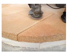
With a handsaw trim around the perimeter of the floor tiles cutting the calcium silicate board flush to the tiles ..
