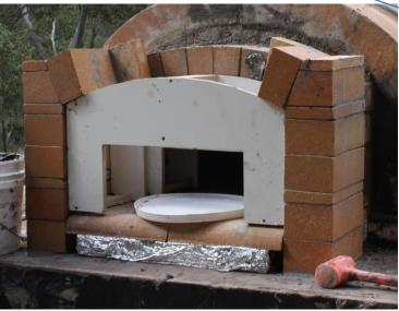
Please start off by DRY laying your front floor tiles including the UF1 and 2 then place your template with the spacer/packer under each point of the template. This will be easier to pull the template out at a later stage.
