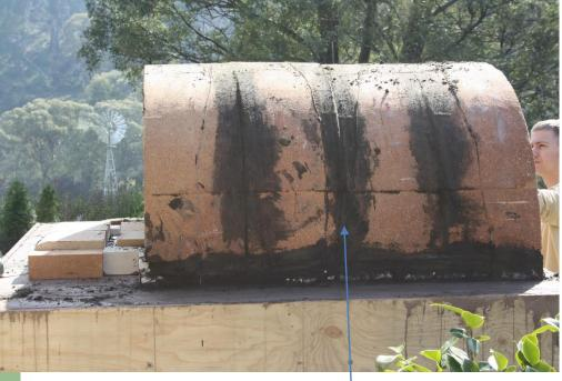
Make sure you have filled in all the gaps in between the joins putting a thin layer of mortar not thicker than 2mm – If the gaps do appear larger you can use the ciment fondu. Mix this 1 part Fondu and 3 parts washed sydney sand and fill into joints
