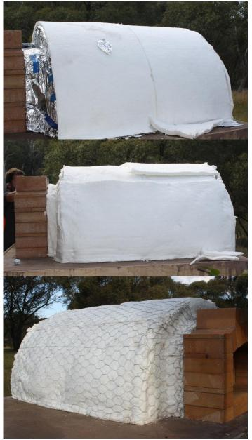
Ceramic insulation blanket can be irritable And a dust mask an gloves must be worn when handling this product....
