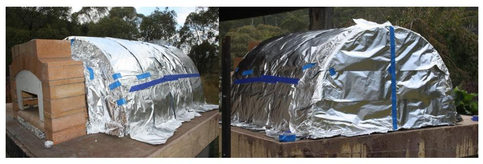
• Before you attempt to insulate the oven wrap the ovens chamber in Aluminium foil like a hot potato. You can do 1 layer or 5 layers the more the better. This stops the water from getting into the chamber.
